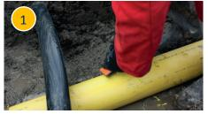
Using a marker pen, mark the position of Anaconda's tapping tee on the main and prepare the pipe surface area with a pipe scraping tool
