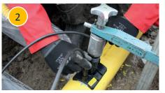
Clamp the tapping tee onto the prepared main using the correct clamping force. Fuse the tapping tee using the fitting's welding parameters
