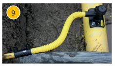
The connection is now complete. The installation should be pressure tested before commissioning.
