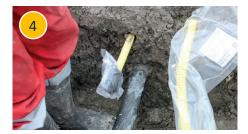
Place the fitting on the service pipe and push fully up to the insertion depth. Keep the packaging on the fitting to protect from contamination
