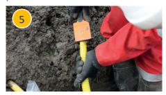
When the tapping tee is fully cooled, prepare Anaconda's pipe spigot. Mark the fitting's insertion depth
