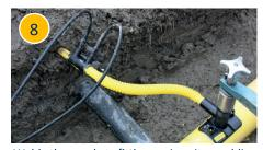
Weld the socket fitting using its welding parameters. Once the fitting is fully cooled, remove the clamps
