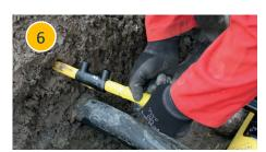
Fully insert Anaconda's prepared pipe spigot into the fitting up to the insertion depth
