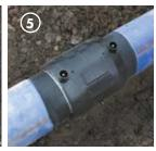
Prepare the pipe ends following the ProFuse® pipe preparation for electrofusion jointing above. Follow industry best practice and water industry procedures to make the joint and cleanse and test the pipeline.
