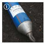
Attach the towing head directly to the leading end of the pipe coil. This operation is undertaken without removing the CleanPipe™ seals, located internally, a short distance from the pipe ends.
