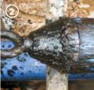
The pipe remains sealed throughout the whole installation procedure. Contamination from the installation process remains outside the factory seal.
